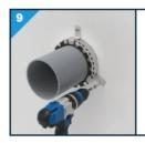
Distribute the remaining Multiclips proportionally and secure with screws.
